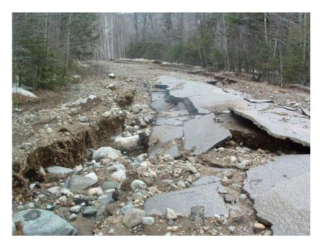
Figure 41. Route 120 Washout in Andover Caused by Blocked Culvert, Maine April 5, 2005
