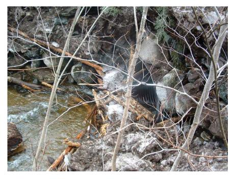
Figure 42. Route 120 Washout in Andover Caused by Blocked Culvert, Maine April 5, 2005
