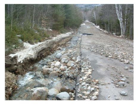
Figure 43. Route 120 Washout in Andover Caused by Blocked Culvert, Maine April 5, 2005
