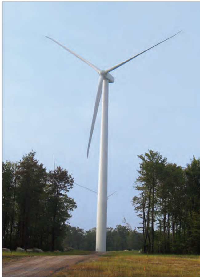
Figure 2. A wind turbine shown in a “feathered” position during the curtailment experiment at the Casselman Wind Project in Somerset County, south-central Pennsylvania.
