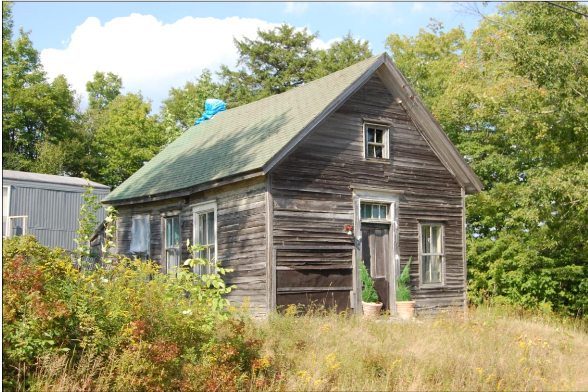
Photograph 13. Former School, 660 Sugar Hill Road, Eastbrook (Survey Map No. 68).
