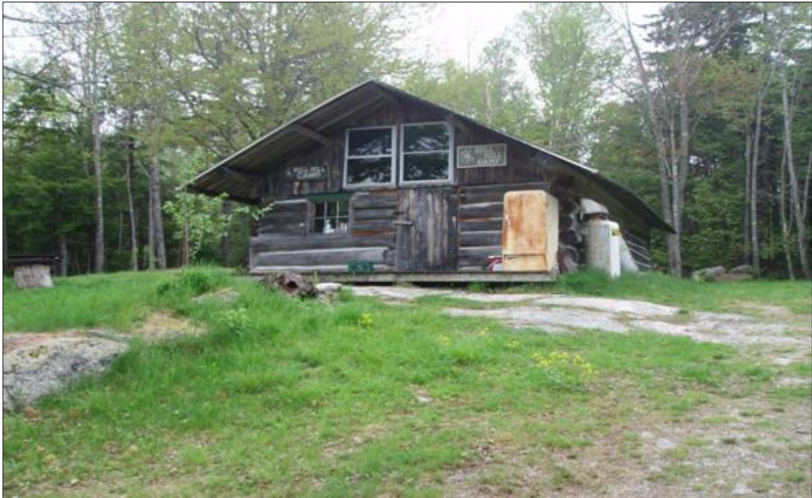
Photograph 1. Bull Hill Camp, this contemporary camp building is located within one-mile of the turbine locations and will remain in this location.
