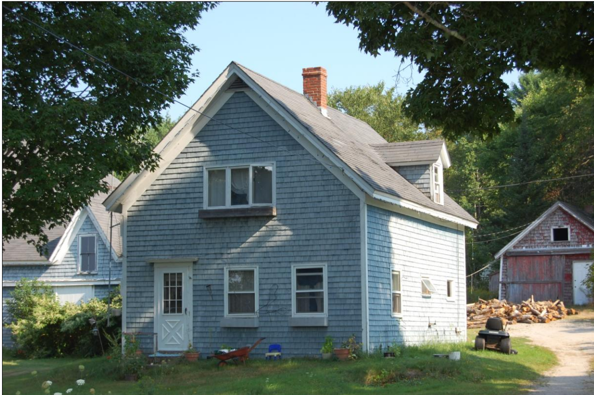
Photograph 9. House, 118 Eastbrook Road/Route 200, Eastbrook (Survey Map No. 33).
