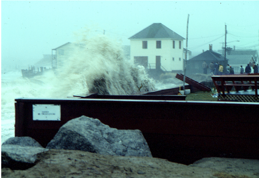
Storm wave impact on a wooden sea wall at Camp Ellis in Saco. Photo by S. M. Dickson.
