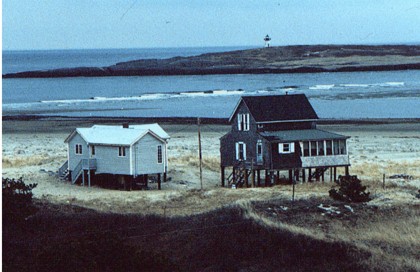
Two homes on Hunnewell Beach that were damaged by erosion and flooding and subsequently moved landward and elevated on posts. Photo by S. M. Dickson.
