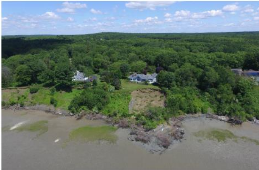
Figure 6. An oblique aerial photograph of the March 2016 landslide at Bunganuc Bluff. The slope failed east of the 2013 landslide shown in Figure 3. June 30, 2016 photo courtesy of Rick Harbison, GPCOG.
