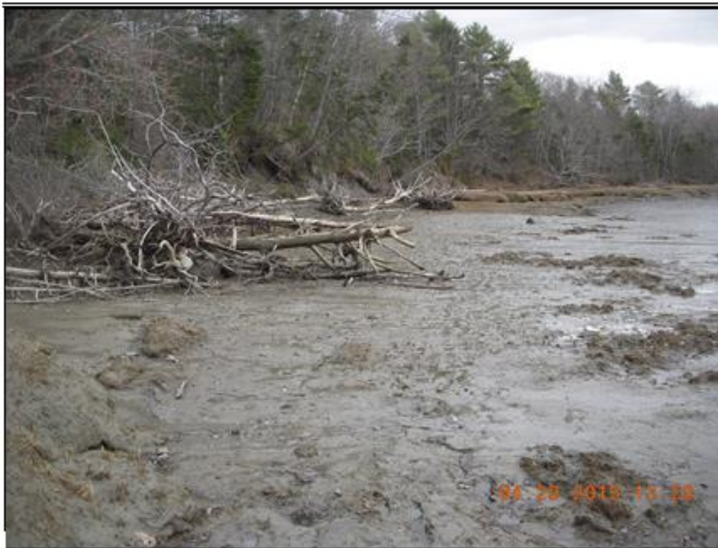
Figure 1. This photograph shows the Miller Point shoreline in the vicinity of the project area. Unstable slopes (Bryant et al. , 2002) of Presumpscot Formation mud experience slope failures that lead to drift logs on the upper intertidal profile and sediment platforms that become colonized with salt marsh vegetation. Fringing marshes exist in the foreground (lower left) and distance. These marsh segments are experiencing erosion as part of a natural cycle. Eroded sediment is contributed to the adjacent mud flats. MGS file photo by S. M. Dickson, April 29, 2015.
