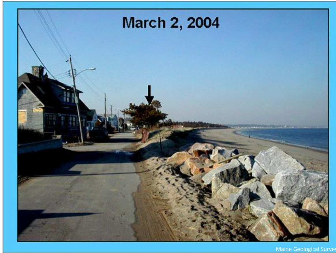
Photograph from March 2, 2004 of end of seawall.
