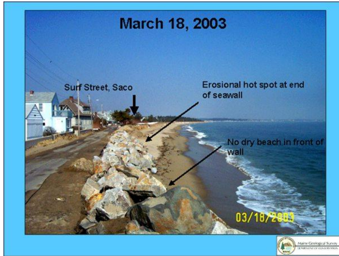
Photograph from March 2003 showing erosional hot spot at end of seawall.
