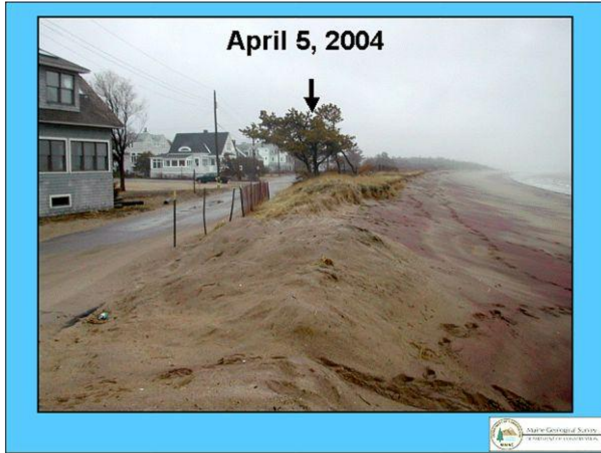
Photograph from April 5, 2004 showing overwash of fill area onto Surf Street.
