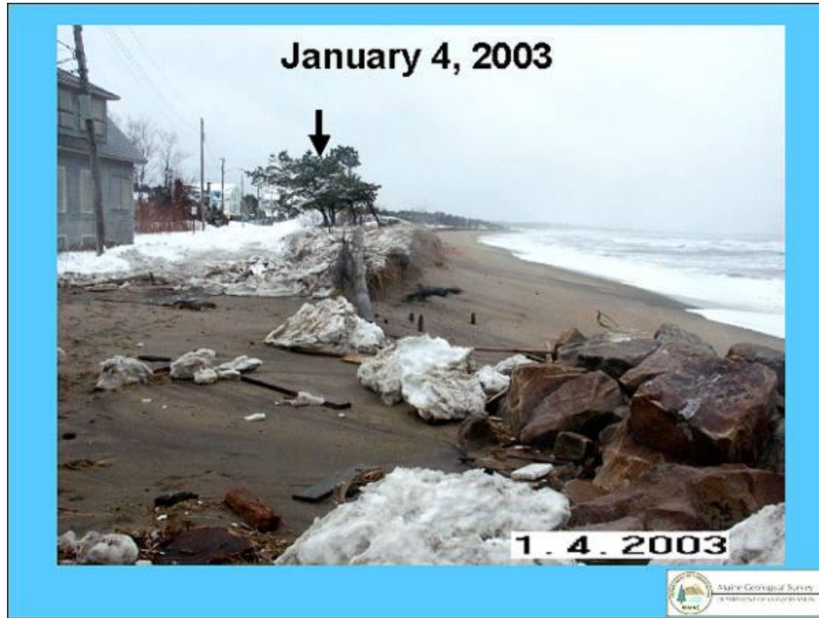
Photograph during January 2003 northeast storm showing erosion and overwash of the artificial fill area, and erosion of natural dune area north of the seawalls.
