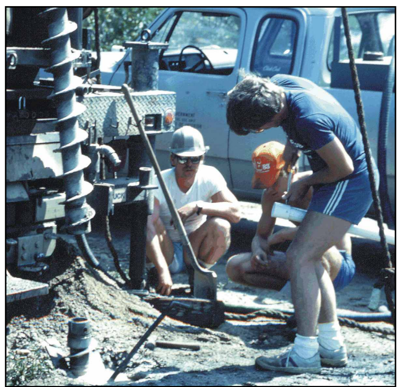
Installing a monitoring well, Washington County, Maine.
