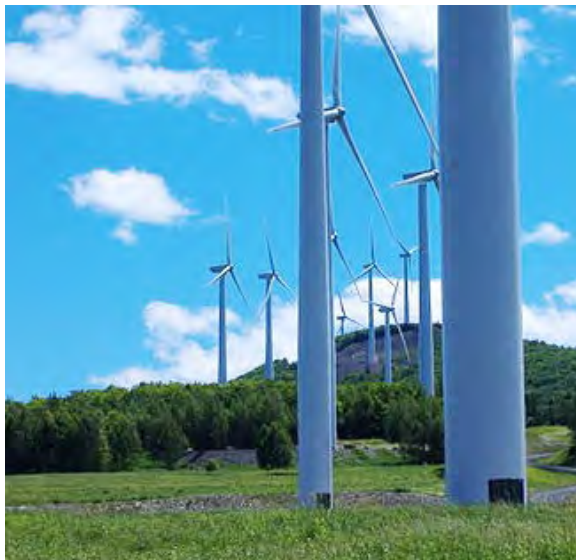
Several of the twenty-eight 1.5 MW wind turbines
