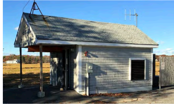
Pump Station #12, King's Highway. Photo: Wright-Pierce.
