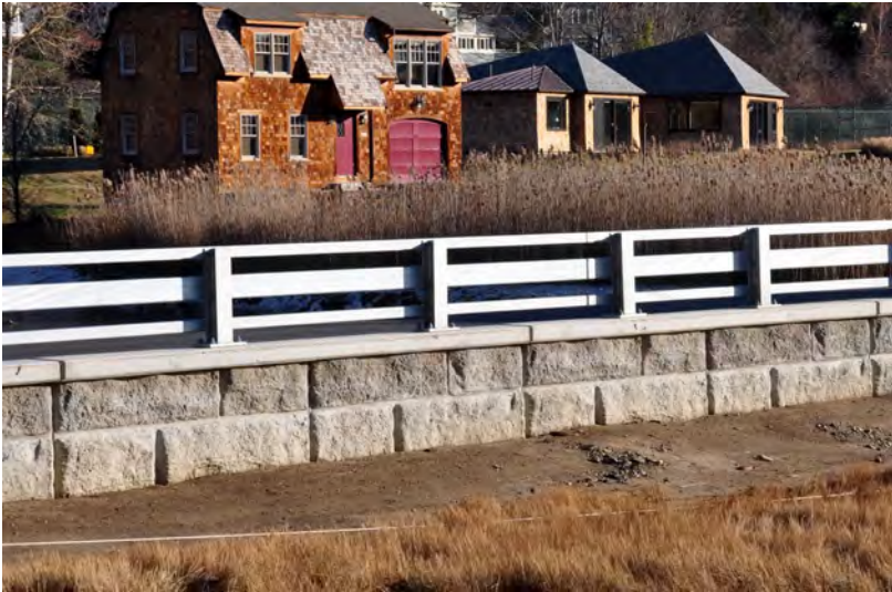
Village Seawall. Photo by Tom Morgan.
