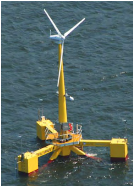
Photo: University of Maine’s Advanced Structures & Composites Center
