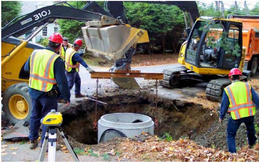
Stormwater drainage and sidewalk construction on North Street. Photo courtesy of the Public Works Department.
