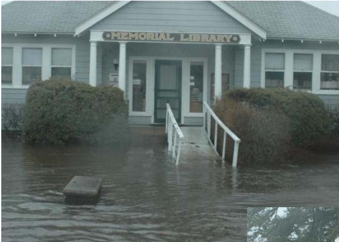
Memorial Library 2-3 feet flooding
