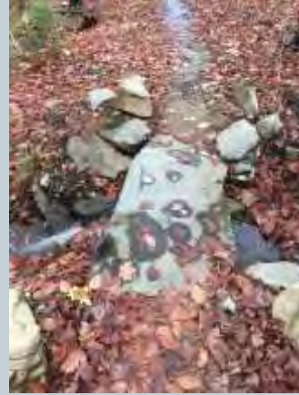
Drainage work on trail
