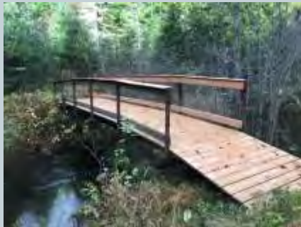
Bridge across Stratton Brook
