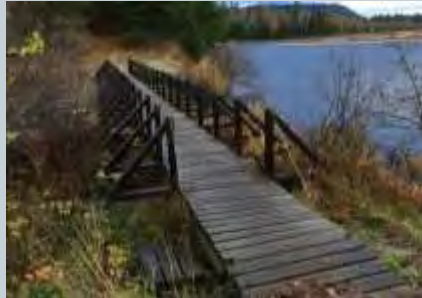
New pedestrian bridge at Stratton Brook Pond Outlet
