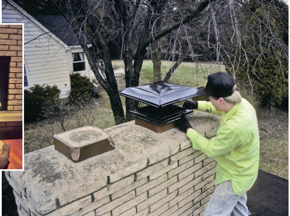
After visually inspecting the chimney to make sure it is clear, install a chimney cap to keep raccoons and other pests out.
