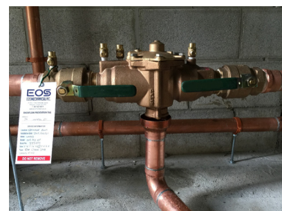
A testable backflow prevention device
