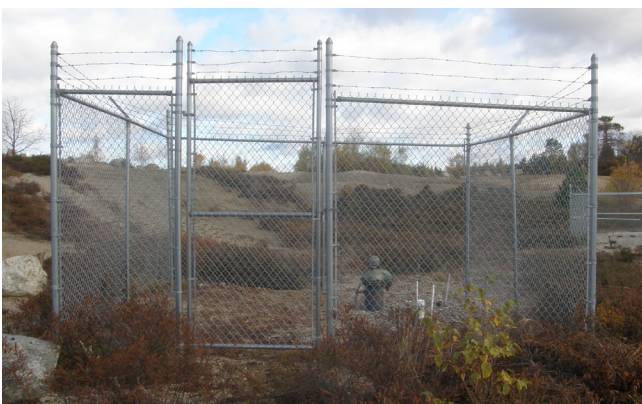
Security fence with locked gate around wellhead.
