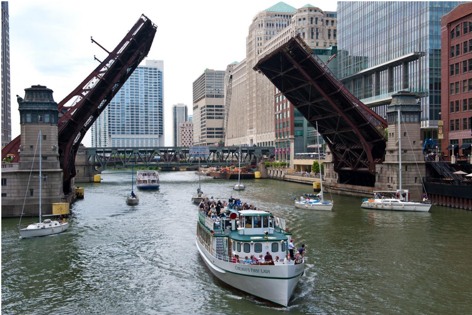
Movable bridges open to let boats through and close to let cars go across.
